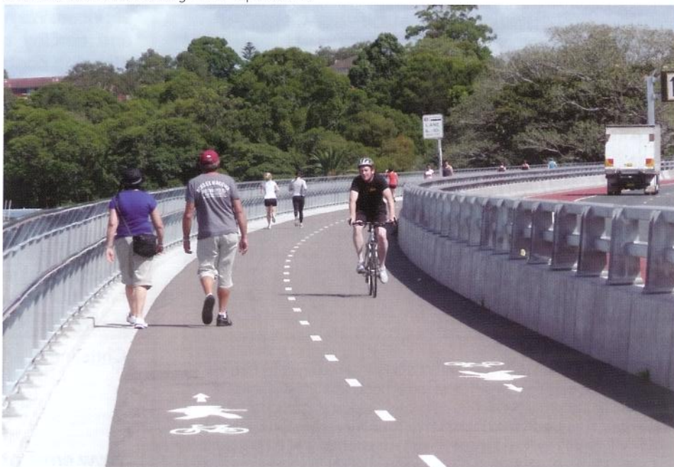
Good quality shared paths are essential infrastructure for a walkable environment
