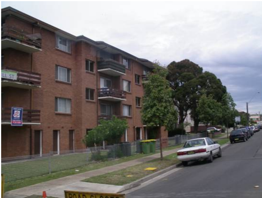
Figure 13: Typical 1970s walk-up flats in Fairfield – note poor quality open space and little low level access for parents and children to open space
