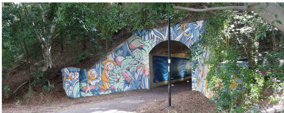
The GreenWay comprises different types of shared paths – this one is part of a former road bridge (Source: Author)
